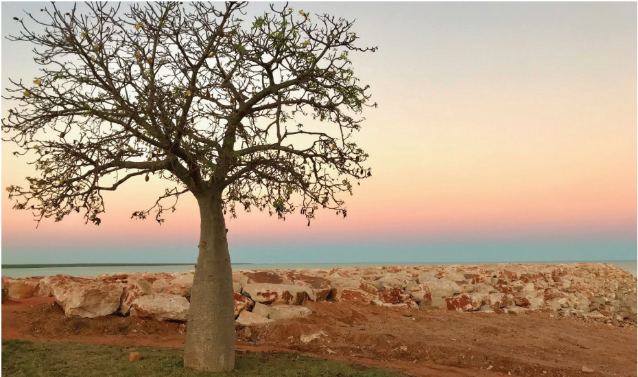
New revetment works along the foreshore. Image: Sarah Taylor-Fuller
